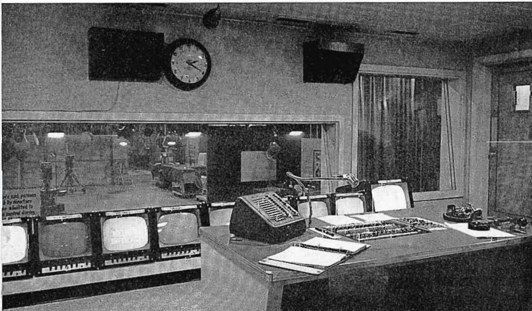
FIG. 8. Production control room. Elevated 5 feet above the studio floor, the director utilizes a row of TM-7 Monitors for program sources. The lighting control board (described elsewhere) is to the right of the switching desk, and the announce booth to the left. Three systems of intercom are available to the director: the push button type which includes the lounge, property storage and announcer's office as well as operating areas, the microphone ceiling speaker system and the standard headset type. (The latter two are tied together). This method of operation with the video and audio control personnel separated from the director has proven very satisfactory.
