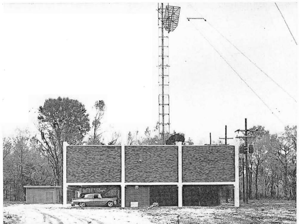
FIG. 16. WWL-TV Transmitter, near city of Gretna some five miles from downtown New Orleans studio, is housed in a modern brick and concrete building of windowless design. Unusual feature is placement of air circulating
